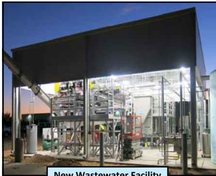
New Wastewater Facility
