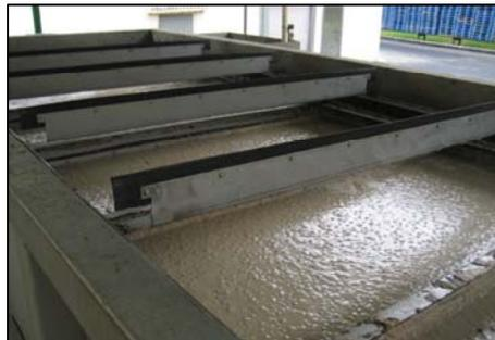
biological pond system for removal of dissolved BOD. Significantly, 100gpm of filtered reuse water is now brought back to the plant.
