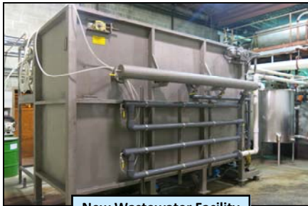
New Wastewater Facility
